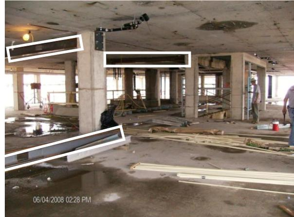
Structural steel reinforcing around stairs and elevator. Piece on lower left to be installed
