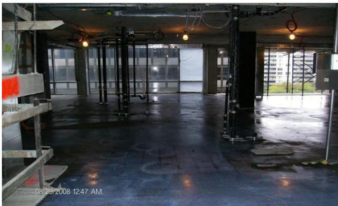
Slab leveling complete after installation of risers creating constructability issues.
